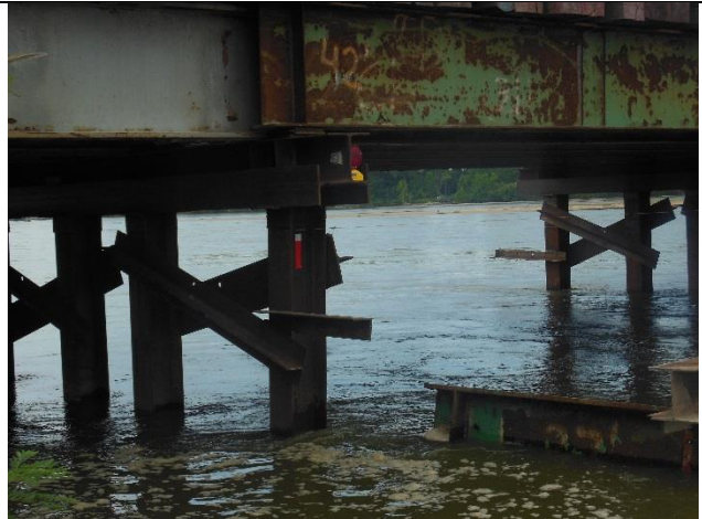
September 4, 2015 – Photo showing flashing light and reflective tape on upstream side of bent row #2.
