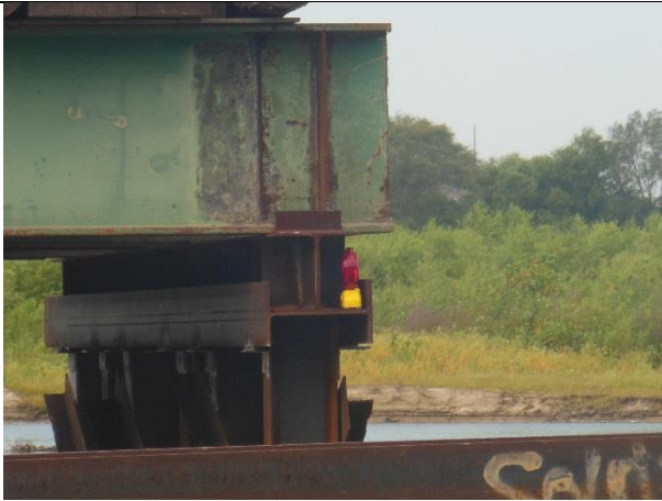
September 4, 2015 – Photo showing flashing light on upstream side of finger #2.
